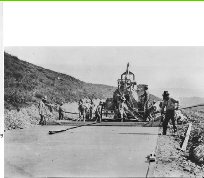
Rolling and Tamping 20'x4" Concrete Pavement 8-
