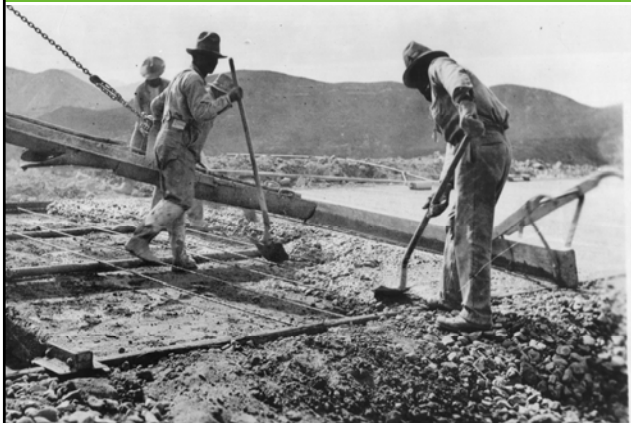
Placing \frac{3}{8} " Sa reinforcing rods in 20'x4" Concrete Pavement 8-7-19
