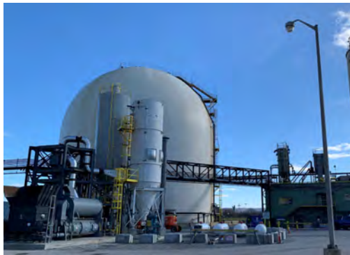
Feed ash drying at 5 tph Separation at 30 tph Equivalent to production fly ash processing
