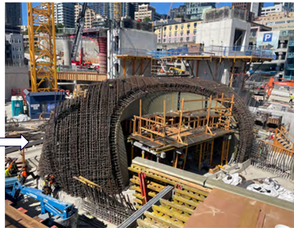
REBAR PLACEMENT ONSITE (INSIDE ZONE C)
