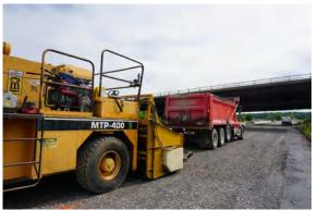
Dump truck drove 15 min to job site Discharged to a spreader then paver
