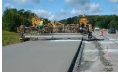
Paving, Curb & Gutter Low slump concrete
