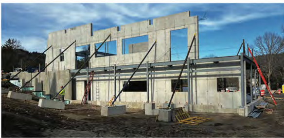
The designers for the DEEP project designed a thermal mass wall utilizing concrete made with post-consumer ground-glass pozzolan cement to optimize the site's solar orientation all year round. The Trombe wall provides passive heating and cooling and improves natural ventilation.
