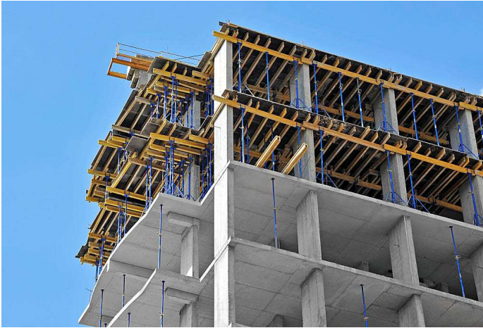
In Situ (Cast-In-Place)
